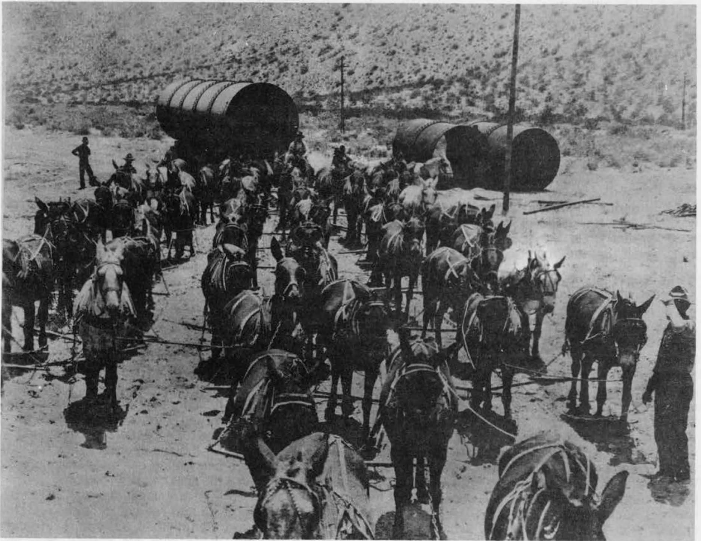
Fifty-two mule teams were used to haul supplies for the aqueduct.
