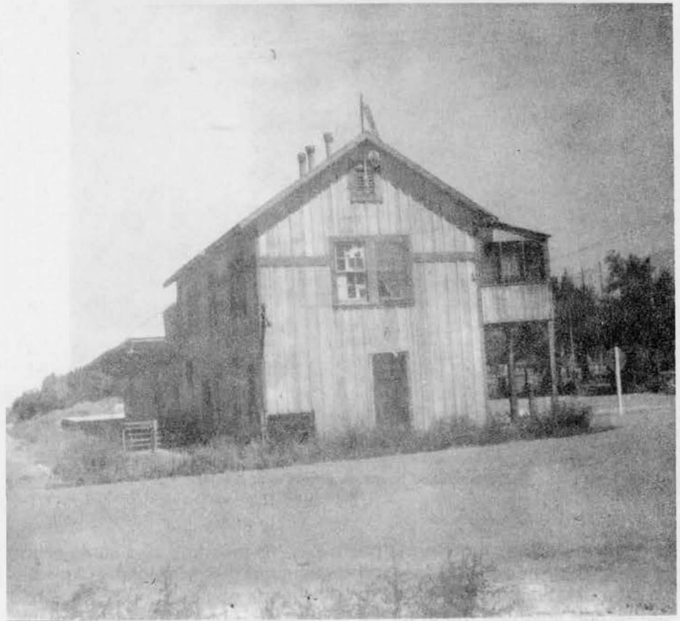
Old railroad station at Keeler.
